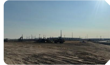
Decommissioned BTC mining and demolished building in Moses Lake
